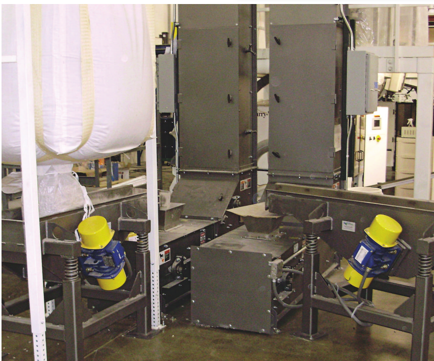
Bulk sacks containing up to 1,300 lb of sunflower seeds, far left, deposit the seeds onto the twin vibratory feeders, which then gently transport them using vibration to a pair of bucket elevators, background. The feeders use a minimum of power.
